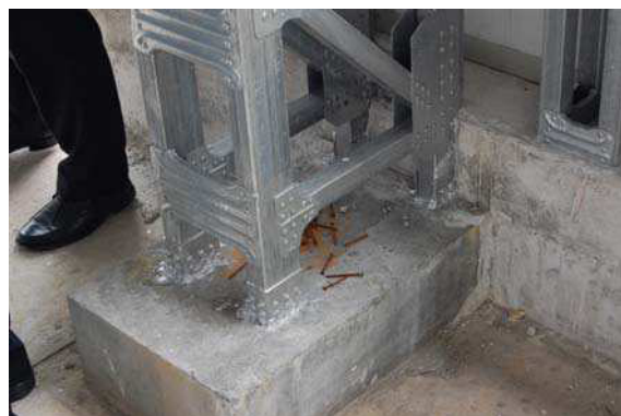
Figure 3 : Effect of corrosion between galvanized steel frame and nails (Exposed to marine environment)
