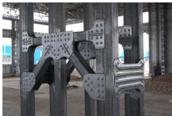
Figure 4 : Connection method between the components
